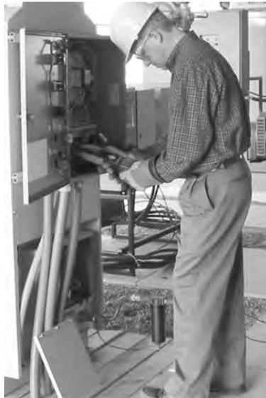
**Figure 5-1—Power line monitor**
