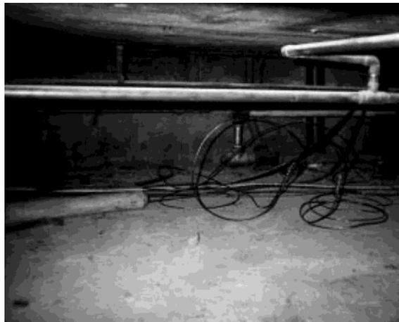
**Figure 11-4—Excessive grounding conductor coil**
