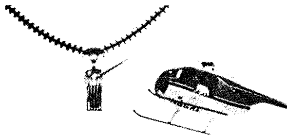
Fig 2 Helicopter Installing Pilot Line
